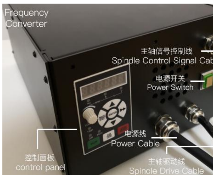
Interface diagram of electric control box
